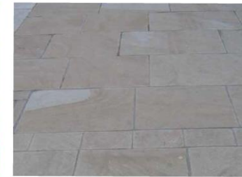
Potential to use the same high quality paving in the garden adjacent to 2-6 Cannon Street and in the garden beside the Abbey to connect the gardens across Distaff Lane
